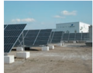
Photovoltaic power plant of RIKEN TECHNOS CORPORATION (within the Gunma Factory site)
