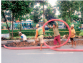
Electric Power Cables
